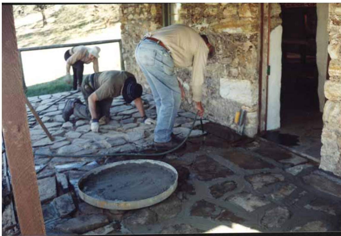
Laying the slate verandah floor – Freeman's Hut
