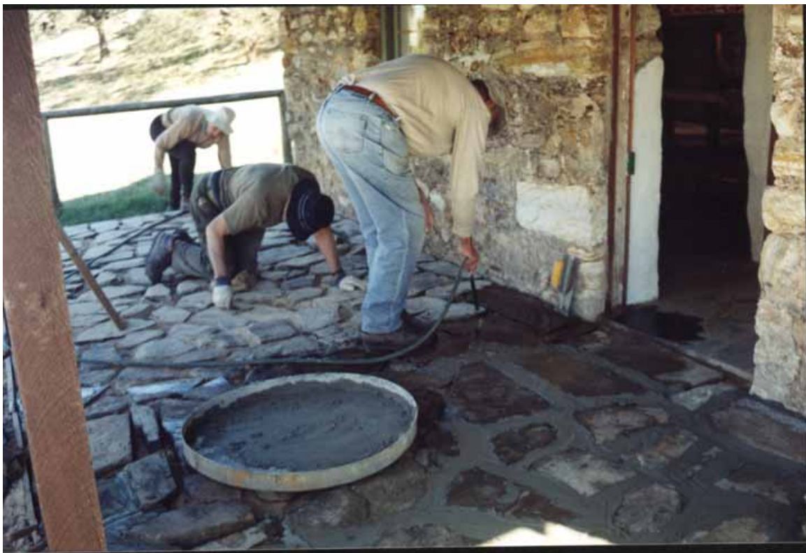
Laying the slate verandah floor – Freeman's Hut
