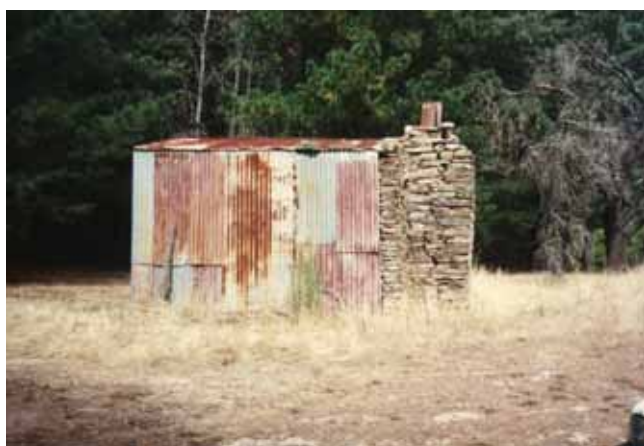
Rossiter Hut, before restoration by the Friends (Doug Leane's team, 1997)
