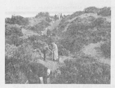
Pictured here are those hard working Friends who constructed the Dutch Sandladder at Waitpinga. Purpose was to reduce the effects of sand movement and damage to the environment. In all 180 metres of ladder were constructed where the Heysen Trail passed from the road to Waitpinga Beach across the sandhills and the River. The project was a great success.
